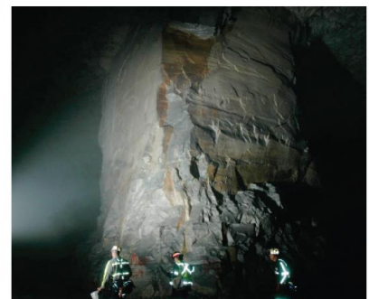
Rib failure due to a joint intersecting the pillar.
