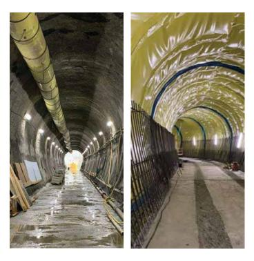
JENNMAR Civil and Turnstone Industrial Solutions are excited to be a part of the design-build Atlanta Plane Train Tunnel West Extension Project at Hartsfield-Jackson Atlanta International Airport, where JENNMAR Civil supplied lattice girders, bolts, and shaft ground support products to reinforce the terminal and sky train above.Turnstone Industrial Solutions LLC. supplied ventilation and tunnel liner.
