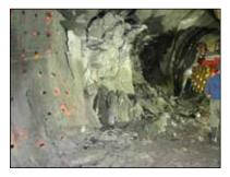
stone, concrete and reinforced concrete. "Dā-mite is mixed with water and placed in the appropriately placed predrilled holes, where it sets and expands, fracturing the rock/concrete". No license required. There are four grades of Dā-mite, providing enough versatility to be utilized in drilled hole diameters from 1 in. to 2 % in.
