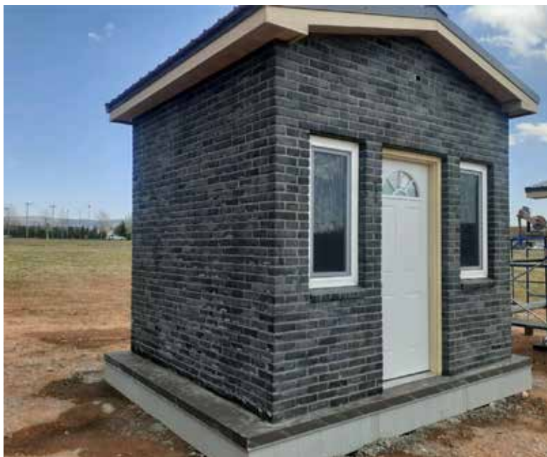
A demonstration house made of materials from coal was built at the University of Wyoming campus.
