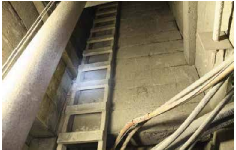
Montana Tech's UMEC, secondary escapeway.
