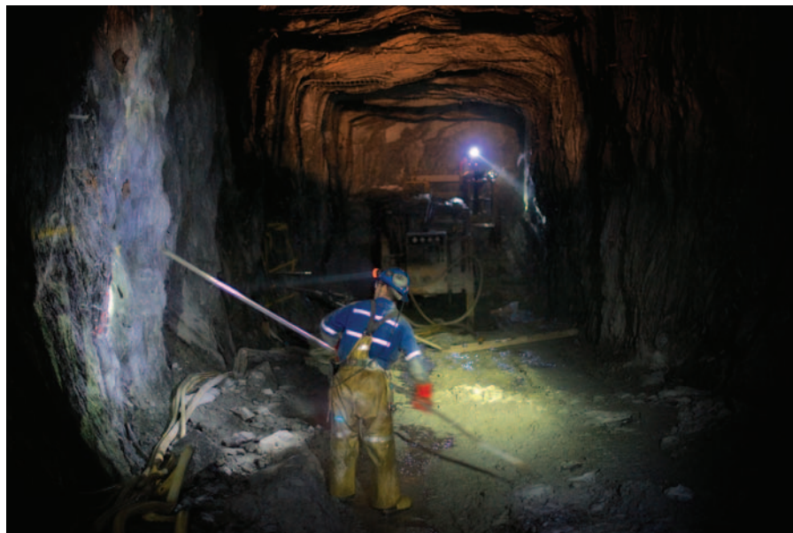
Scaling work at Lake Shore Gold's Bell Creek Mine in Sudbury, Ontario. Photos courtesy of the Ontario Ministry of Northern Development and Mines.
