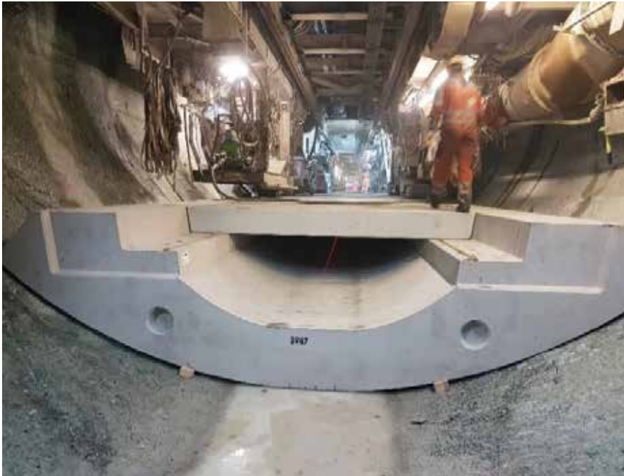
Precast concrete floor decking for a TBM tunnel.
