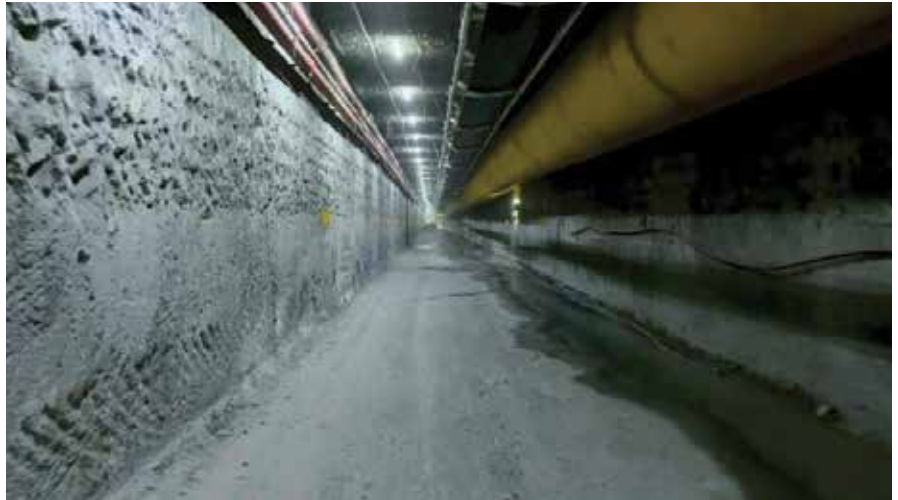
Figure 7 Flat-floor TBM tunnel trial at Fresnillo Mine, Mexico.
