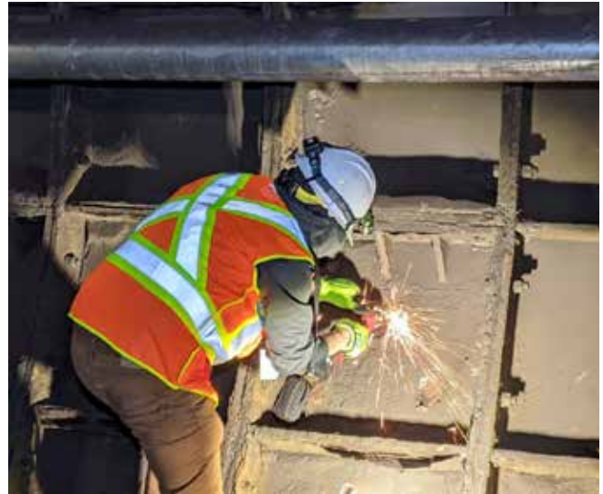
Grinding of steel liner coating for ultrasonic testing of steel tunnel liner at the WMATA Yellow Line project.
