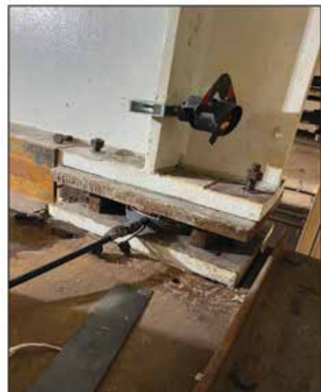
FIGURE 12 Jacking and target point on the header beam.
