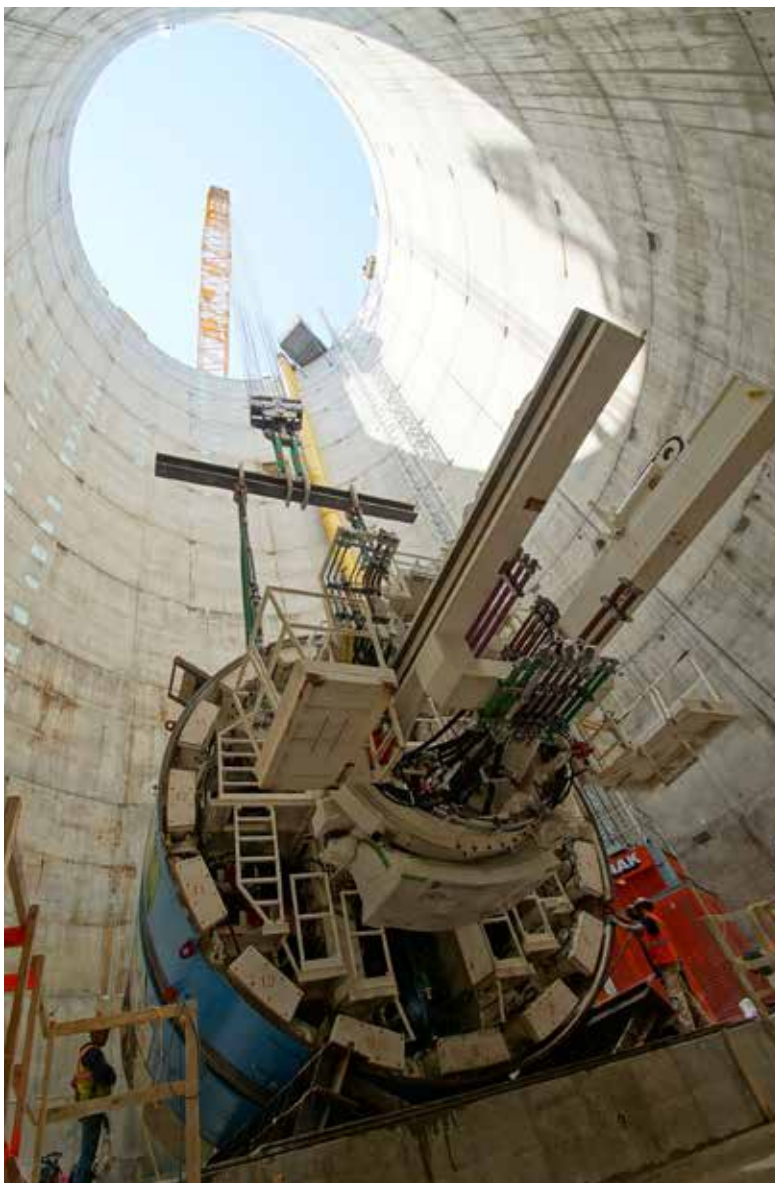
One of the three Herrenknecht TBMs used at the Washington Clean Rivers Project. Herrenknecht remanufactures TBMs at its plant in Kehl, Germany.
