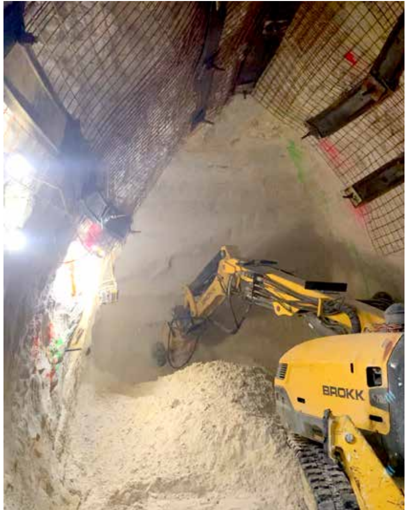
The drum cutters — or road headers — with the Brokk 520Ds meticulously shaved away the sandstone and shale to precisely meet the template shape.
