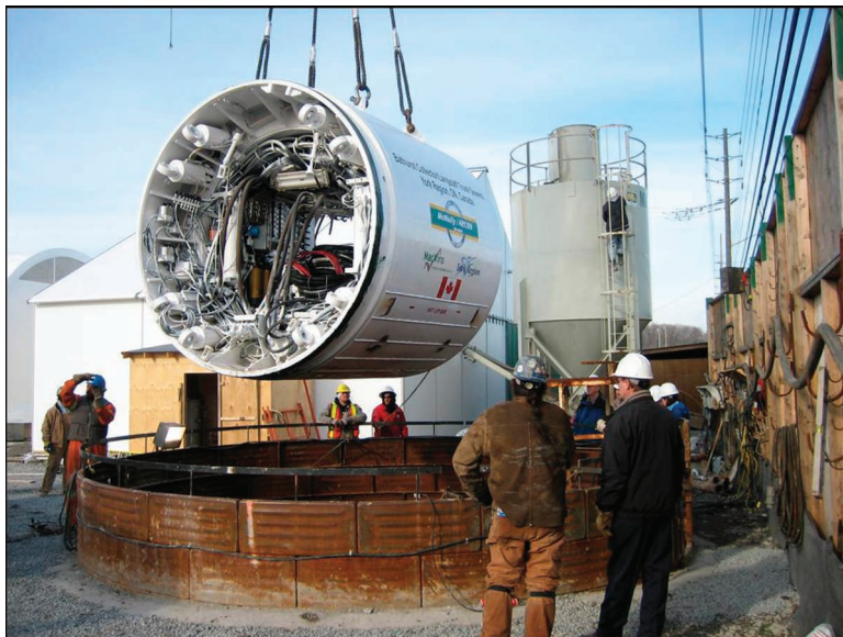
TBM installation at the C7 Shaft for Bathurst South Drive.
