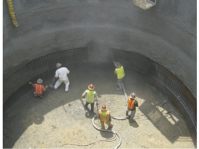
Applying shotcrete at the School Street shaft.
