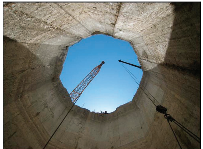
Completed slurry wall shaft on the 19th Avenue tunnel drive.
