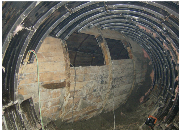
The 2.6-m (102-in.) tunnel connection to the mainline 3.6-m (144-in.) tunnel.
