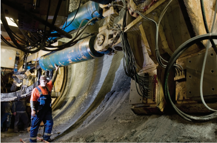
The 6.7 m (22 ft) diameter Robbins Main Beam Machine broke through its first heading on September 29th.
