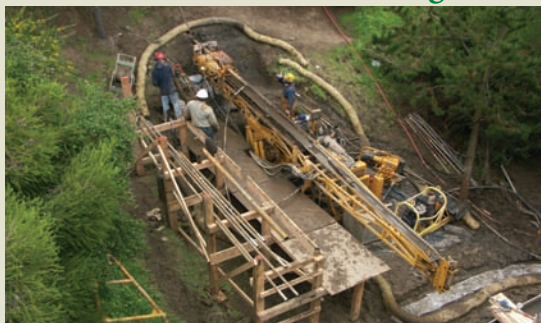
Horizontal Coring for Tunnel Investigation
