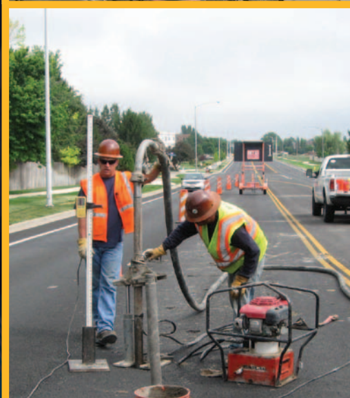
Jet Grouting — Brightwater Conveyance System, Seattle, WA
