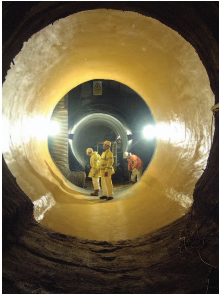
Workers inspect a tunnel sprayed with a waterproofing membrane.
