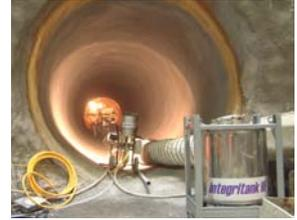
Innovative solutions are available for the external waterproofing of cut and cover and immersed tube tunnels as well as for the waterproofing of suspended decks in all tunnel types. The latest addition to the Company's range is the Integritank HF sprayed waterproofing membrane, which enables owners, designers and contractors to effectively waterproof the internal linings of SCL/NATM tunnels, and can be non-destructively tested to confirm 100% integrity.
