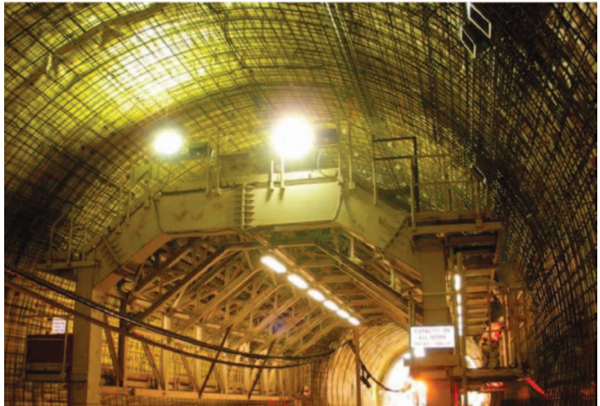
Service gantry at the Devil's Slide Tunnel project.
