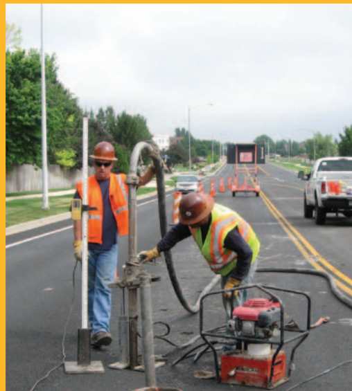
Jet Grouting — Brightwater Conveyance System, Seattle, WA
