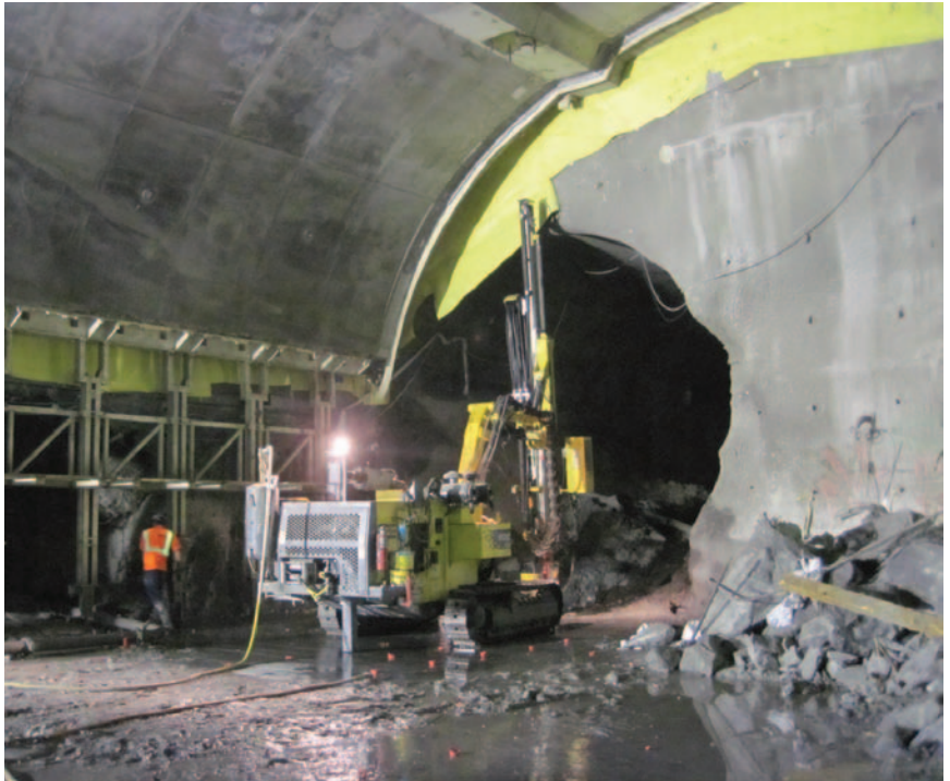
Drilling blastholes in westbound cavern.
