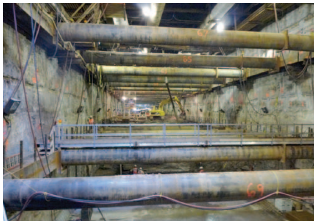
Permanent slurry wall downstage bracing.
