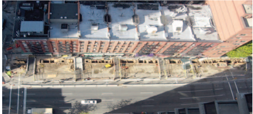
Relocation of utilities adjacent to the west side of Second Avenue.
