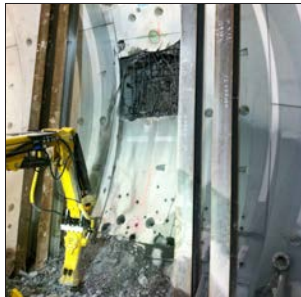
The Brokk 400, equipped with a hydraulic breaker, knocked out chunks of the concrete casing in one of the main traffic tunnels to begin one of the five cross passages in the POMT project.
