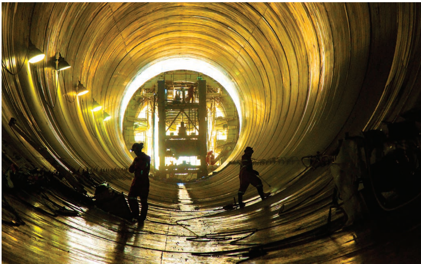
The Waneta Expansion Project in Trail, British Columbia included the construction of two penstock tunnels.
