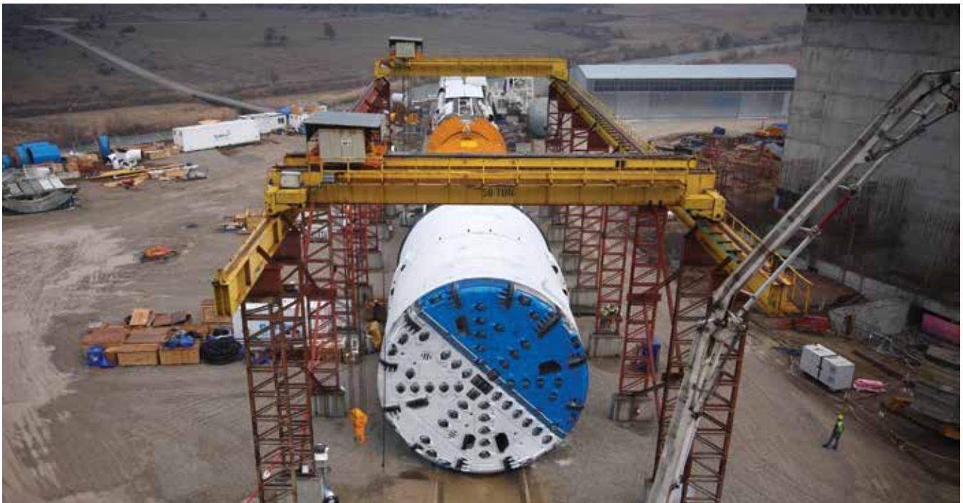
Double shield TBM for Kargi.
