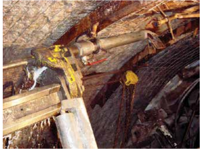
Drilling through stand pipe at Parbati.
