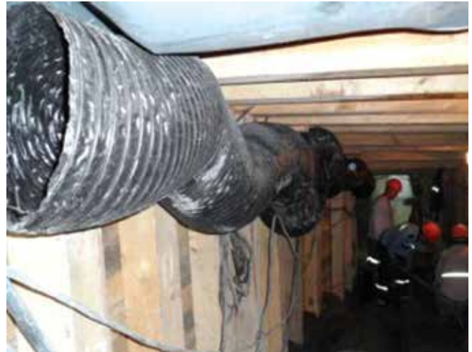
Bypass tunnel excavation.
