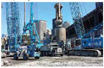
lands comprised of decades of undocumented fills, debris, and various organic deposits. Within the upper reaches of the soil profile, numerous timber piles and railroad ties from buried trestles can be expected. The various fill deposits overlie soft and loose marine sediments that lie on top of glacial till at depths of 12 to 27 m (39 to 88 ft).
