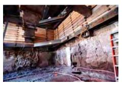
Jet grout cut-off for installation of the Mulry Square vent plant.  $\label{eq:continuous} % \begin{subarray}{ll} \end{subarray} % \begin{subarra$
