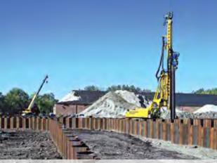
Sheet piles for a cut and cover CSO tunnel.
