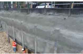
Temporary soldier piles and lagging for earth retention to facilitate tunnel construction.
