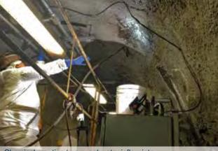
Chemical grouting to prevent water inflow into a subway tunnel.
