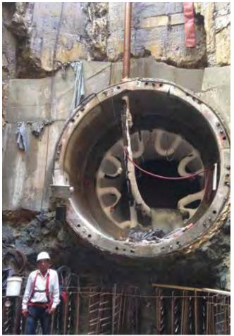
Access Shaft 3, the intermediate shaft located between the launch shaft and the treatment plant, experienced persistent leaks during initial excavation attempts.
