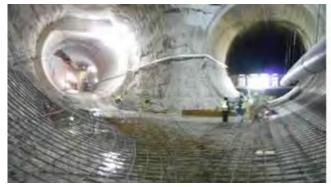
The existing nominal 305-mm (12-in.) thick unreinforced concrete liner was scribed with a radial saw cut at the limits of replacement that are established by the structural engineer's inspections and evaluation of field and lab test results.
