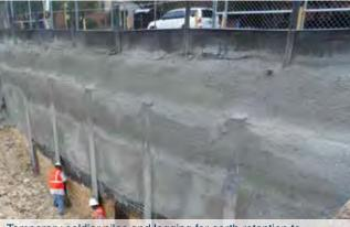
Temporary soldier piles and lagging for earth retention to facilitate tunnel construction.
