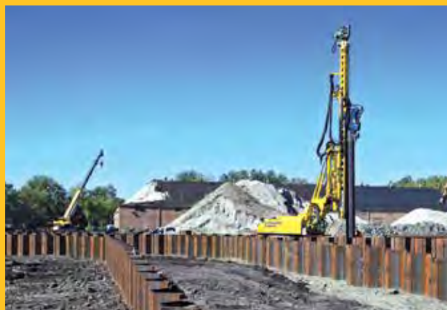
Sheet piles for a cut and cover CSO tunnel.
