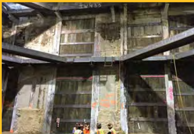
Chemical grouting and jet grouting for excavation support in an urban subway tunnel.
