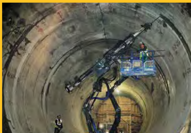
Drilling and grouting for water control around a CSO tunnel.
