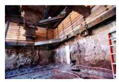
Jet grout cut-off for installation of the Mulry Square vent plant.
