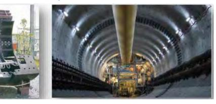
TBM is equipped with an air lock system and saturation diving shuttle which allowed hyperbaric intervention as needed. Seven hyperbaric interventions with up to 10.8 bars were implemented during the tunneling operation. Figure 9 shows tool replacement under atmospheric pressure.
