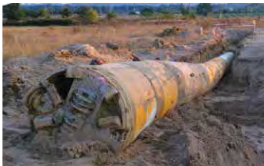
On Oct. 12, 2016, the AVN800 achieved the last of two breakthroughs in Czeszów, Poland using the direct pipe method.
