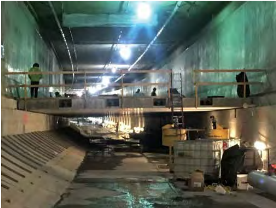
Crews were working on the lower deck of the SR-99 tunnel that will carry traffic northbound through the tunnel. Photo by William Gleason.
