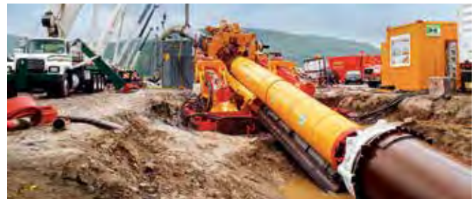
River crossing realized with the Herrenknecht Direct Pipe technology
