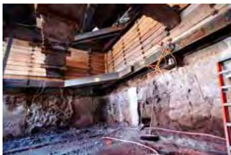
Jet grout cut-off for installation of the Mulry Square vent plant.
