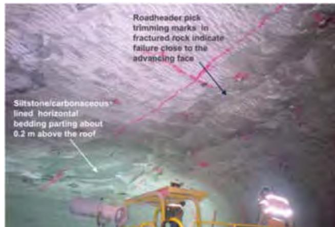
7 for a low friction bedding parting located at about 0.5 m (1.6 ft) above a 7 m diameter (23 ft) tunnel.
