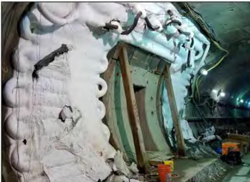
Short haunch freeze pipes were installed through the tunnel liners below the springline of both tunnels to freeze just beyond the limits of the excavation. Although a shadow did not exist above the tunnels, it was decided that haunch freeze pipes would also extend above the springline of the tunnels instead of drilling additional freeze pipes from the ground surface.
