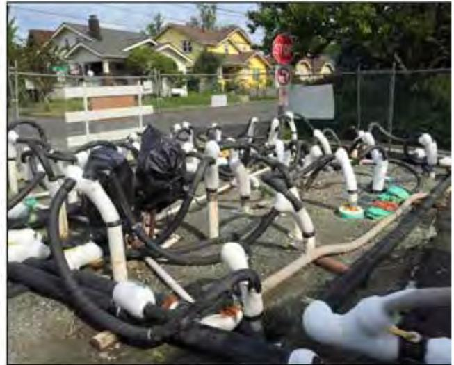
Where there were no utilities located within the freeze grid, ground movement was not controlled and any deformation was repaired as part of the site restoration.
