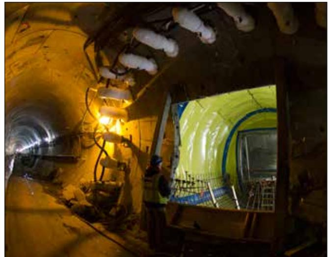
Northgate Link Extension, Seattle, WA, ground freezing for groundwater control and support of excavation
