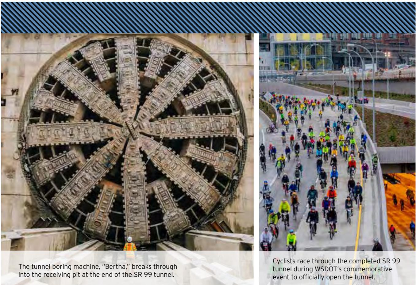
The tunnel boring machine, "Bertha," breaks through into the receiving pit at the end of the SR 99 tunnel.
