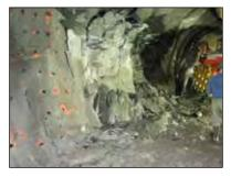
stone, concrete and reinforced concrete. "Dā-mite is mixed with water and placed in the appropriately placed predrilled holes, where it sets and expands, fracturing the rock/concrete". No license required. There are four grades of Dā-mite, providing enough versatility to be utilized in drilled hole diameters from 1 in. to 2  $\frac{3}{4}$  in.
