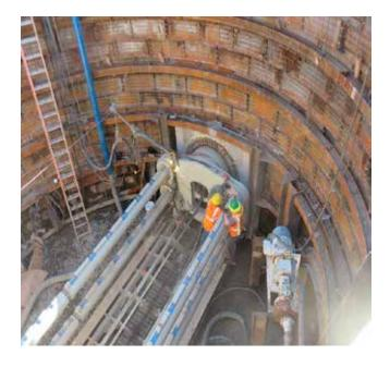
**DSI** - Steel Ribs, Liner Plates, Lattice Girders, Lagging and Miscellaneous Support Items
