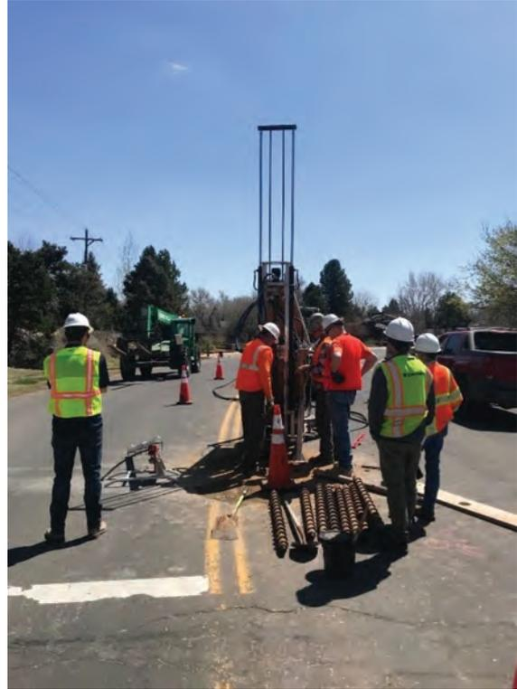
(3-in.) steel casing pipe along the entire length of the newly drilled grout injection points. Pressurized flow was achieved at the existing vent shafts by installing a sewer plug with a bypass hole. The grouting pressure was monitored at the ground surface utilizing a pressure gauge on the injection stack, and the allowable pressure was calculated for each injection point based upon the vertical depth (head) to the HDPE pipe.
