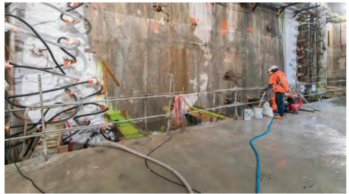
feasibility of ground freezing. The hydrological study showed that flow speeds could be very high locally (20 m/day), which was due to the presence of the fractured Ducey limestone. However, the majority of the fluorescein was not detected even a few weeks after the injection, leading to the conclusion that the average water flow speed (< 0.5 m/day, < 1.6 ftpd) was low enough to practice artificial ground freezing.
