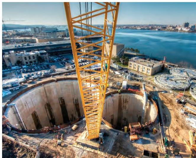
DC Clean Rivers Project, Washington, DC: Division A - Blue Plains Tunnel, reinforced concrete slurry diaphragm wall shafts (pictured); and Division I Diversion Structure, jet grouting for underpinning, support of excavation, and groundwater control
