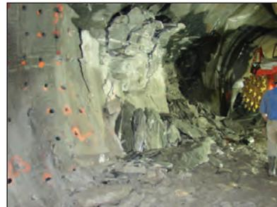
stone, concrete and reinforced concrete. “Dā-mite is mixed with water and placed in the appropriately placed predrilled holes, where it sets and expands, fracturing the rock/concrete”. No license required. There are four grades of Dā-mite, providing enough versatility to be utilized in drilled hole diameters from 1 in. to 2 ¾ in.
