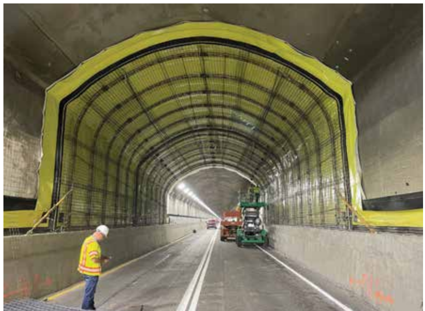
Eastbound tunnel rehabilitation: Membrane and lattice girder installation.
